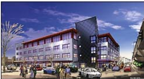
The building, Ballard Lofts, will feature a galvanized steel skin in three colors. One side will feature a black mosaic of interlocking diamond-shaped pieces of steel.
